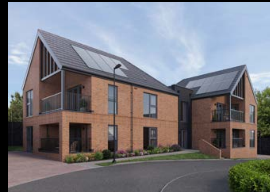
Blackfriars apartments 2 bedroom apartments
